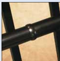
Collar Ring (to cover splice)
