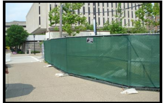
Temporary Fence with Windscreen
