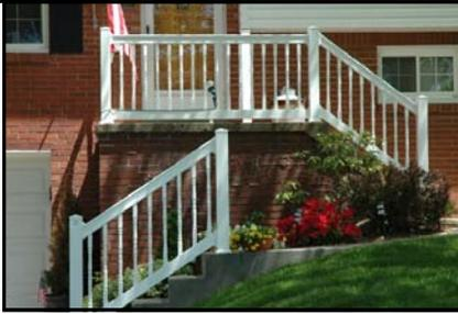
**Vinyl (PVC)** – Polyrail Systems by Digger Specialties provide many options for your vinyl railing including two colors, white and tan. From decorative posts and spindles to the simplicity of square or rectangle rails and pickets, Polyrail Systems is sure to appeal to the most discriminating homeowner. All posts and rails are reinforced for strength and safety. Hidden screws and the bracketed mounting system make it a beautiful choice
