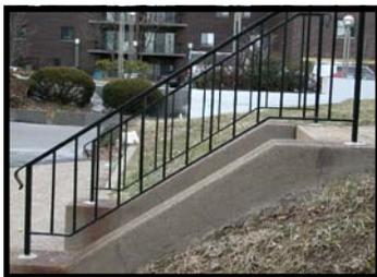
**Welded Steel**—This type of railing is fabricated in our welding shop to fit your exact specifications. Made of solid steel, the railing can be finished with a powder coating, primer paint, or primer and finish paint. Posts are 1" x 1" solid steel with 1/2" x 1/2" solid steel pickets. Posts can be installed in the same fashion as the ornamental aluminum railing.
